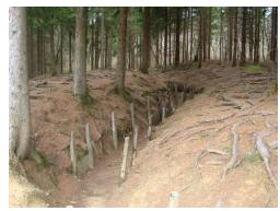
On the left side of this trench, you can see the wood has been stacked to hold back the dirt.
